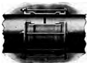
FIG. 60. — Expansion Joint.
